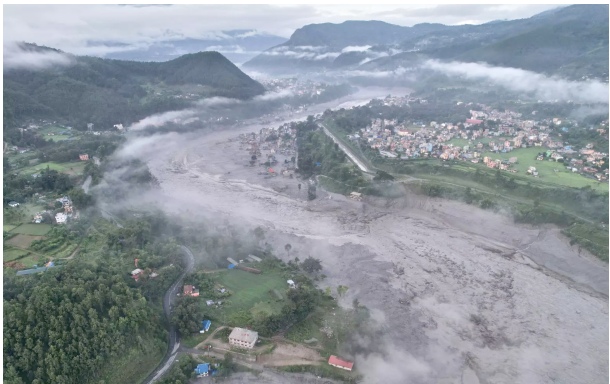
A drone view of the aftermath of flash flooding along the Trishuli river amidst fresh water surge warning in the Trishuli Bazaar area of Nuwakot district, Nepal.
